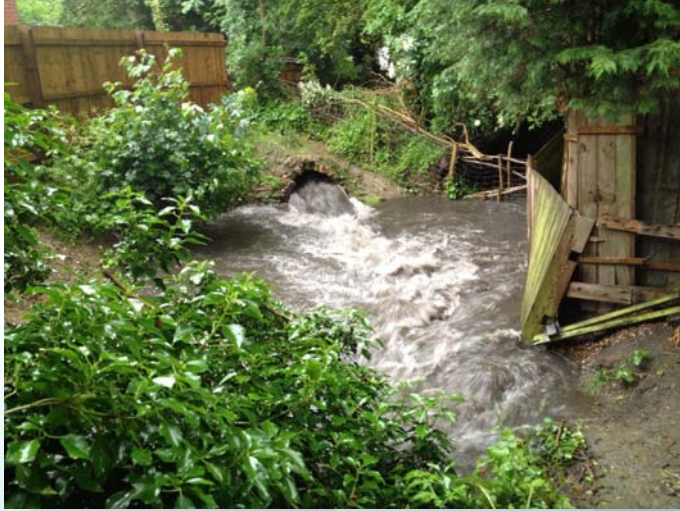
Culvert running full bore
